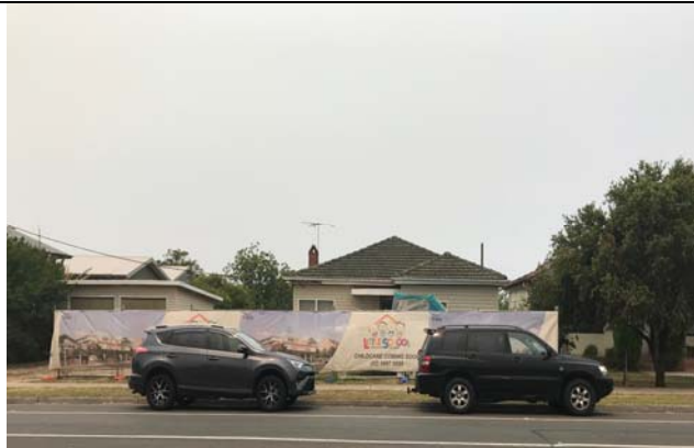
Figure 14 – Child care centre under construction at 331 Blaxcell Street
