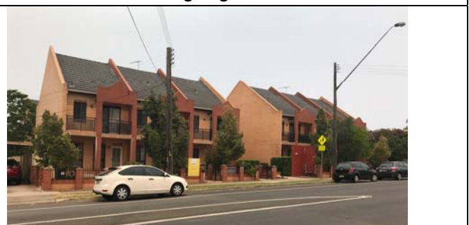
Figure 13 – Multi dwelling development at 335-339 Blaxcell Street
